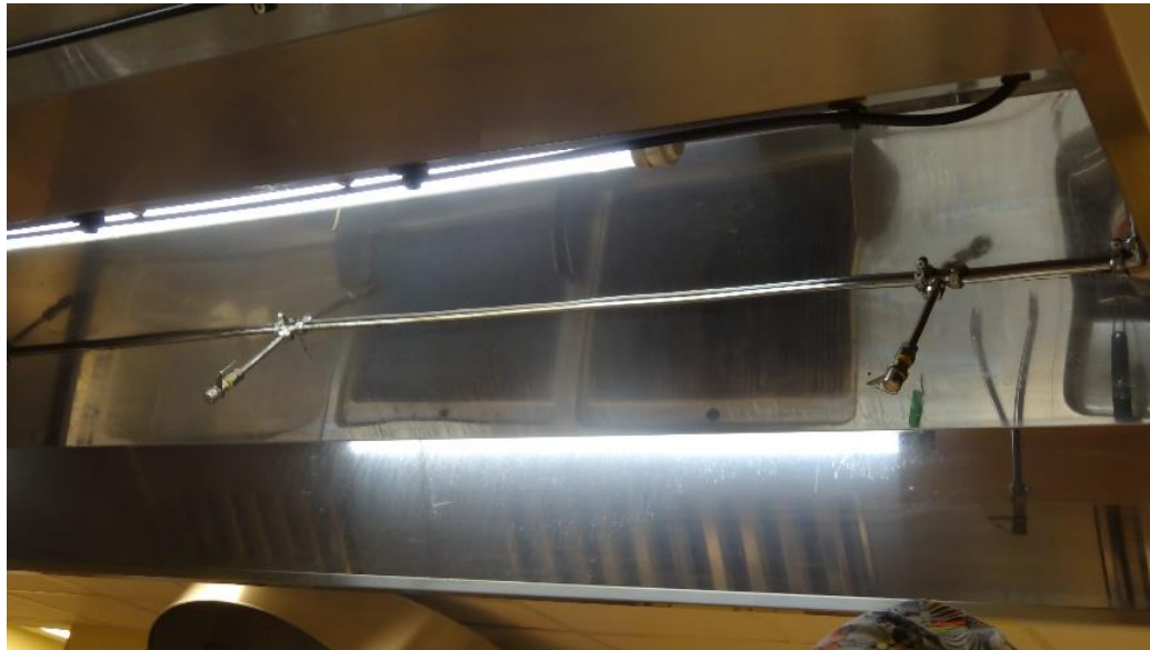
Continuous thermal detection by Easydetect tube
