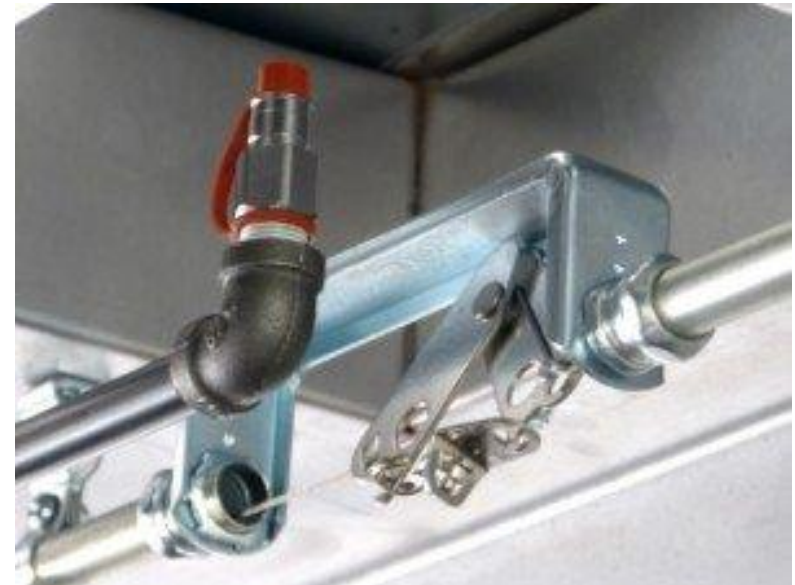
Point detection by thermofusible links
